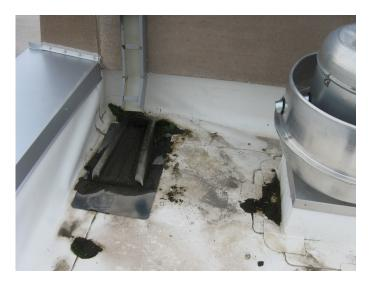
Please refer to LRBP Project Number MR-20 page 42. The Kalispell Armed Forces Reserved Center is approximately 36,000 SF and houses both the MTARNG and the Army Reserves. The single ply (Hypalon) roof was installed in 2004. The roof is beyond economic repair and the replacement is necessary to prohibit further interior damage to the facility. The state share of this project is 36%.
